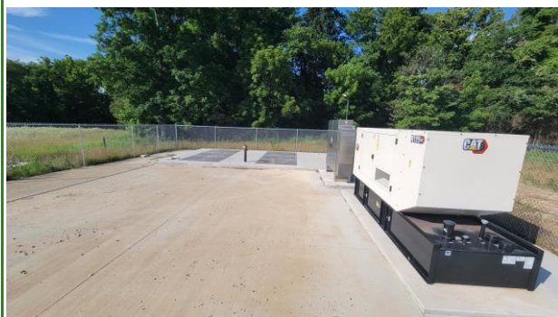
Photo 15 - Sanitary sewer lift station with natural gas emergency generator
