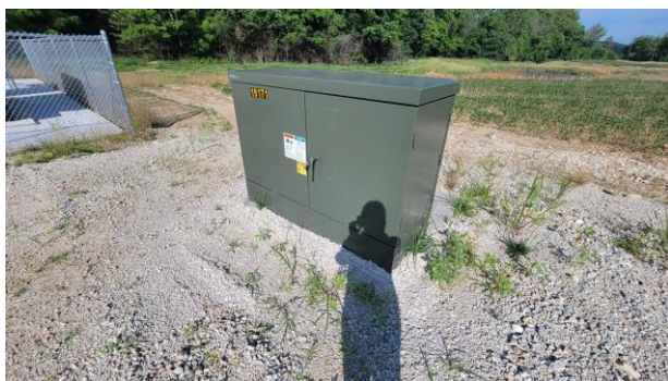
Photo 16 - Pad-mounted transformer associated with the sanitary sewer lift station
